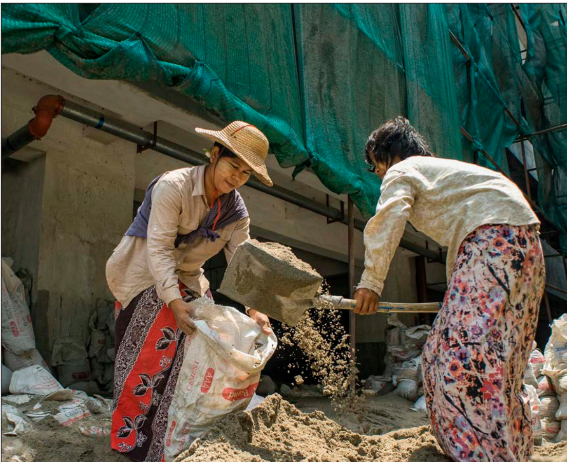
Women moving sand at a construction site in Yangon
