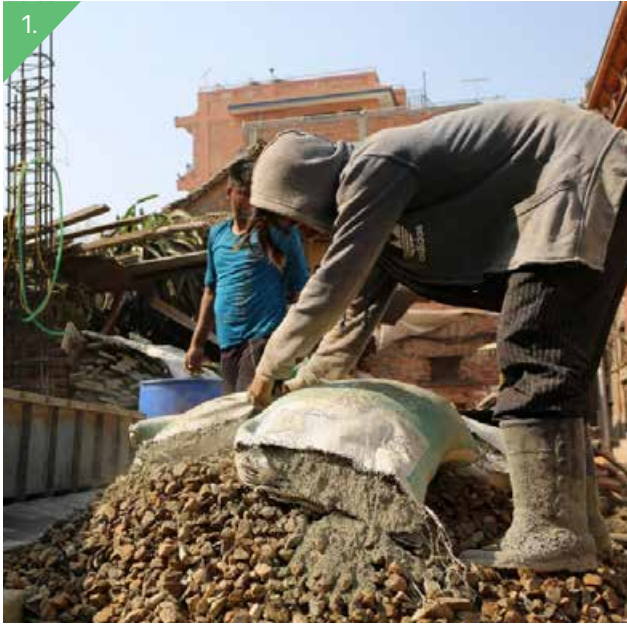
1. Ongoing construction in Bhaktapur, November 2019. Photo: Prabhat R Jha
