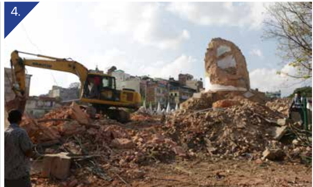
4. An excavator removing debris of Sundhara tower which fell during the earthquake, 2015. Photo: Prabhat R Jha
