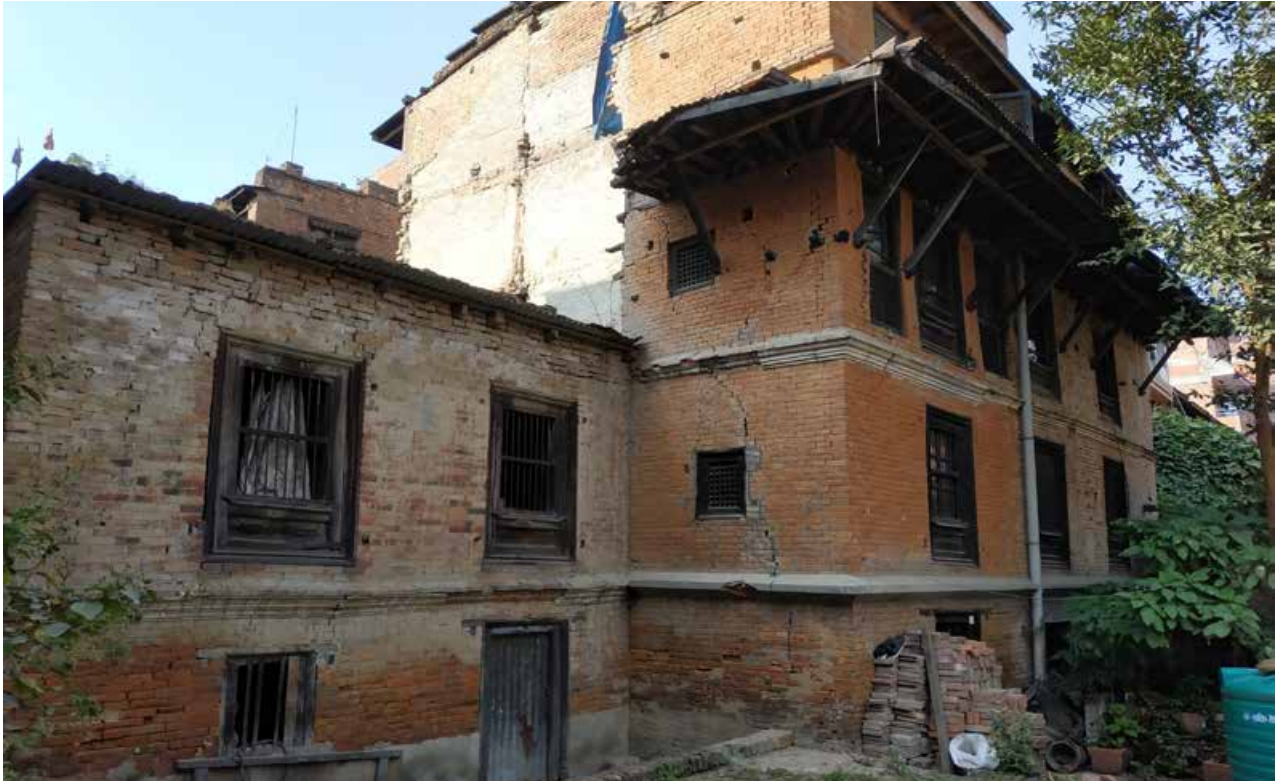
Partially damaged house, Bhaktapur, November 2019. Photo by Lena Michaels
