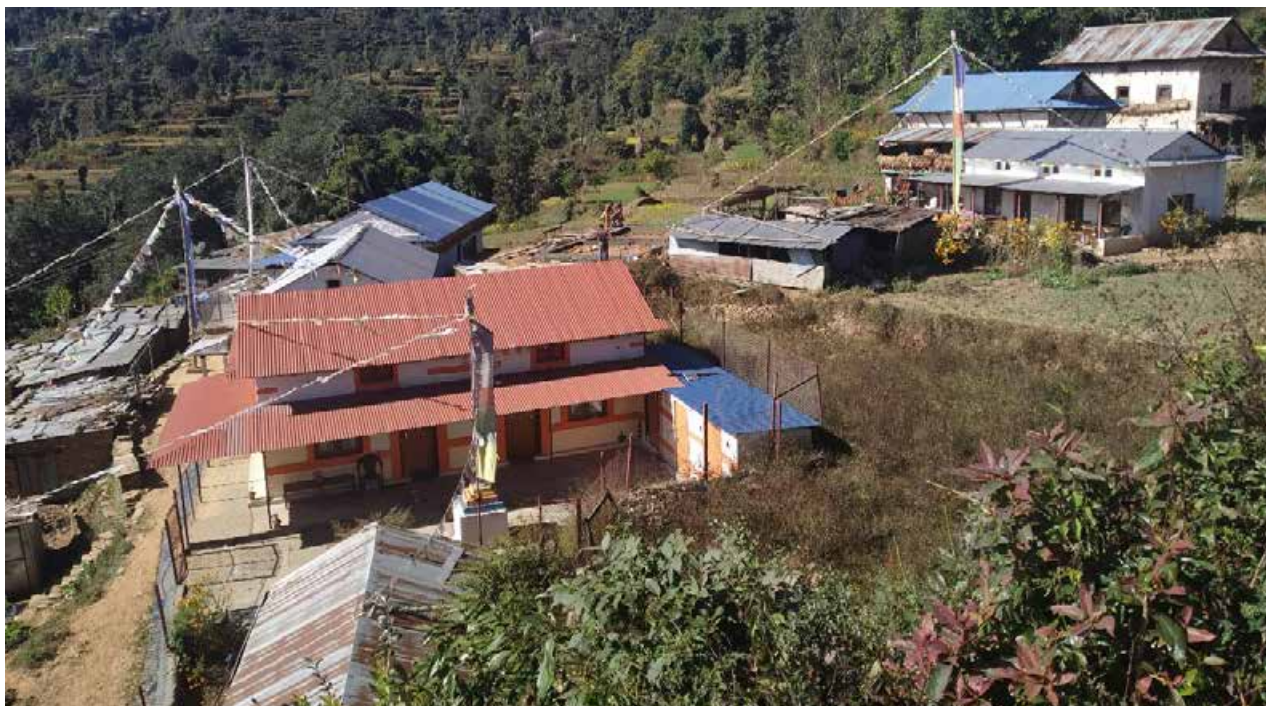
Rebuilt houses in Lisankhu settlement, Sindhupalchok, November 2019. Photo: Aruna Limbu
