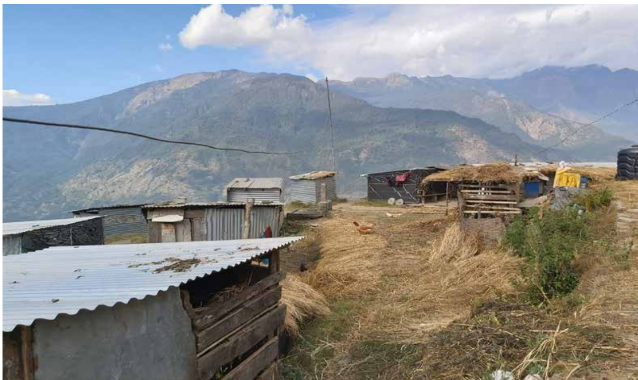
Shelters on government-owned land for a displaced Dalit community in Barpak, Gorkha, 2019. Photo by Manasi Prasai
