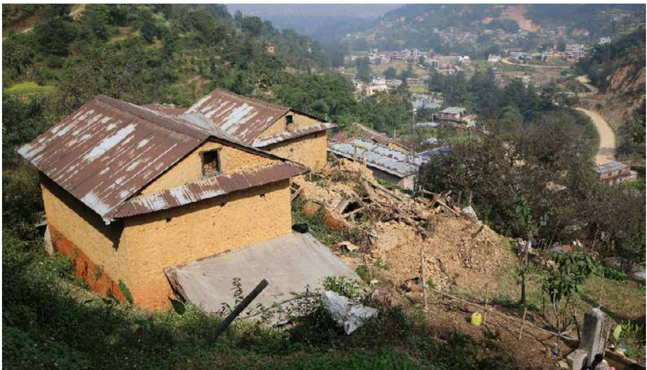
Debris of a house that collapsed during the earthquake, Suryabinayak Municipality, Bhaktapur, November 2019. Photo: Lena Michaels
