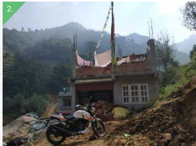
1. A newly built code-compliant house with pillars and rods for future extension, Sulikot Rural Municipality, Gorkha, November 2019. Photo: Manasi Prasai
