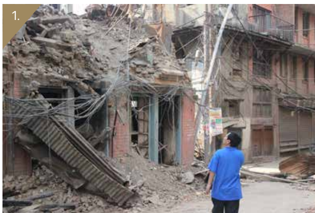
1. Damaged house in Chhetrapati, 2015. Photo by Prabhat R Jha
