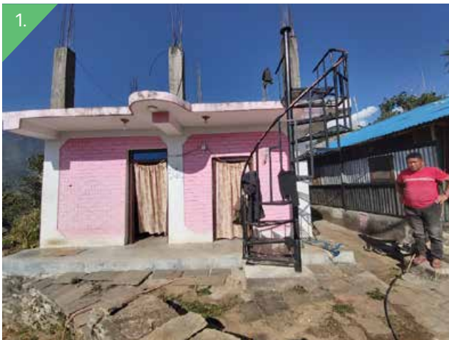
1. A newly built code-compliant house with pillars and rods for future extension, Sulikot Rural Municipality, Gorkha, November 2019. Photo: Manasi Prasai
