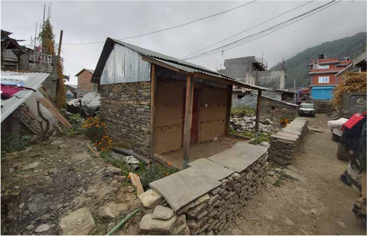
Shop built reusing stones with wood banding in Barpak, Gorkha, 2019. Photo by Manasi Prasai
