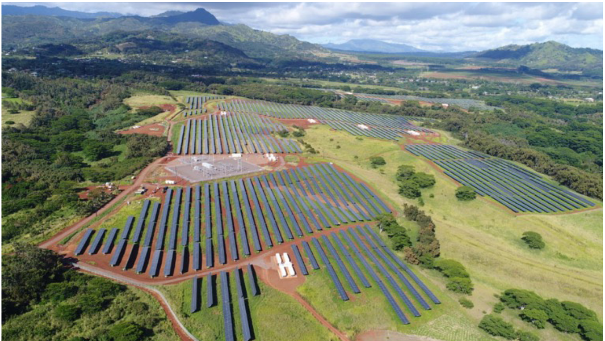
Photo 3. Solar plus battery peaker plant in Kauai, Hawaii.
