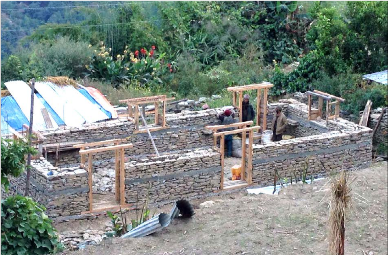
A house rebuilding in Dolakha—Photo: Chiran Manandhar
