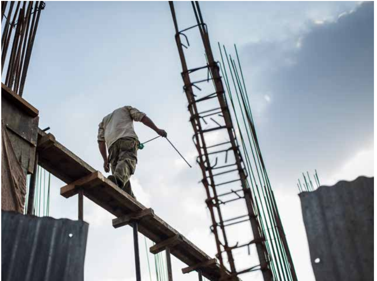
Construction at the new Savar industrial facility in Bangladesh
