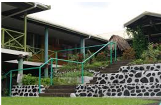
Figure 11. South Pacific Community Education Training Center, Fiji
