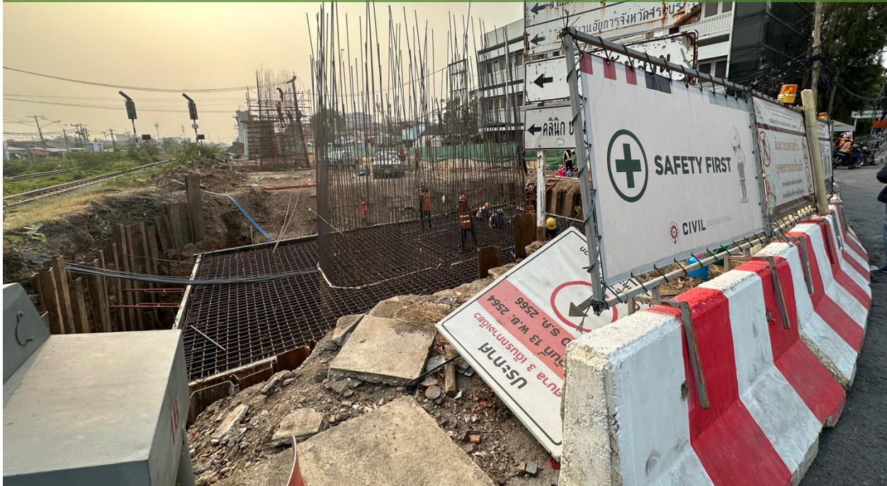
Ongoing construction work in Saraburi, Thailand, for the HSR project.
