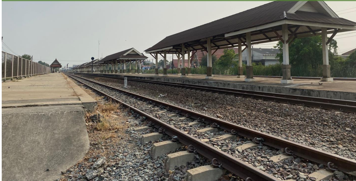
Dual tracks passing through a station in Ayutthaya.
